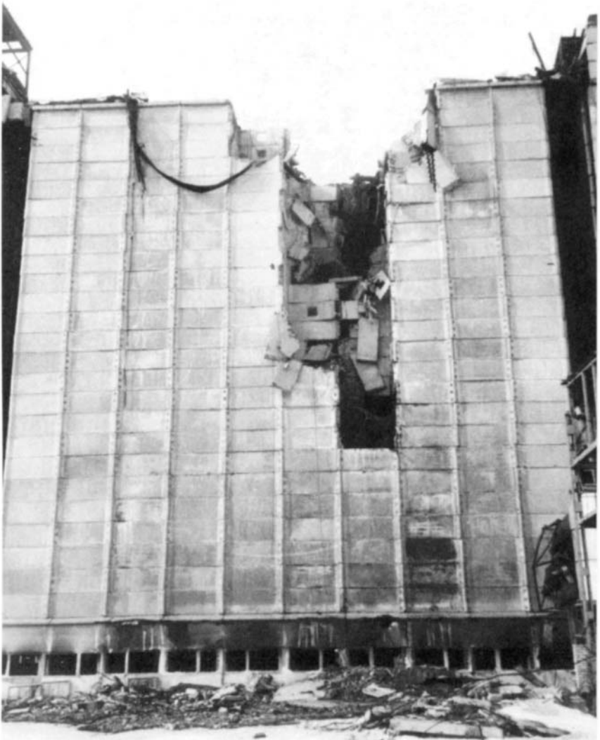
Figure 4-11 The concrete silo complex in Tomylovo, Knibyshev region, Russia that was damaged by a series of smoldering gas explosions in the silo cells. (Courtesy of A. Borisov and B. Gelfand, Moscow, Russia).
