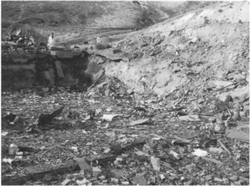
Figure 6-10 Remains of Booster Room 2 of the Sierra Chemical Company Kean Canyon plant east of Reno near Mustang, Nevada, USA, after explosives mix explosion in 1998. From CSB (1998).
