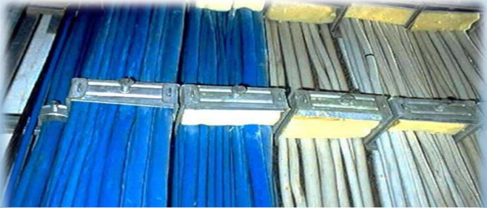
*Ex-ia wiring must be separated from all other wiring.*
